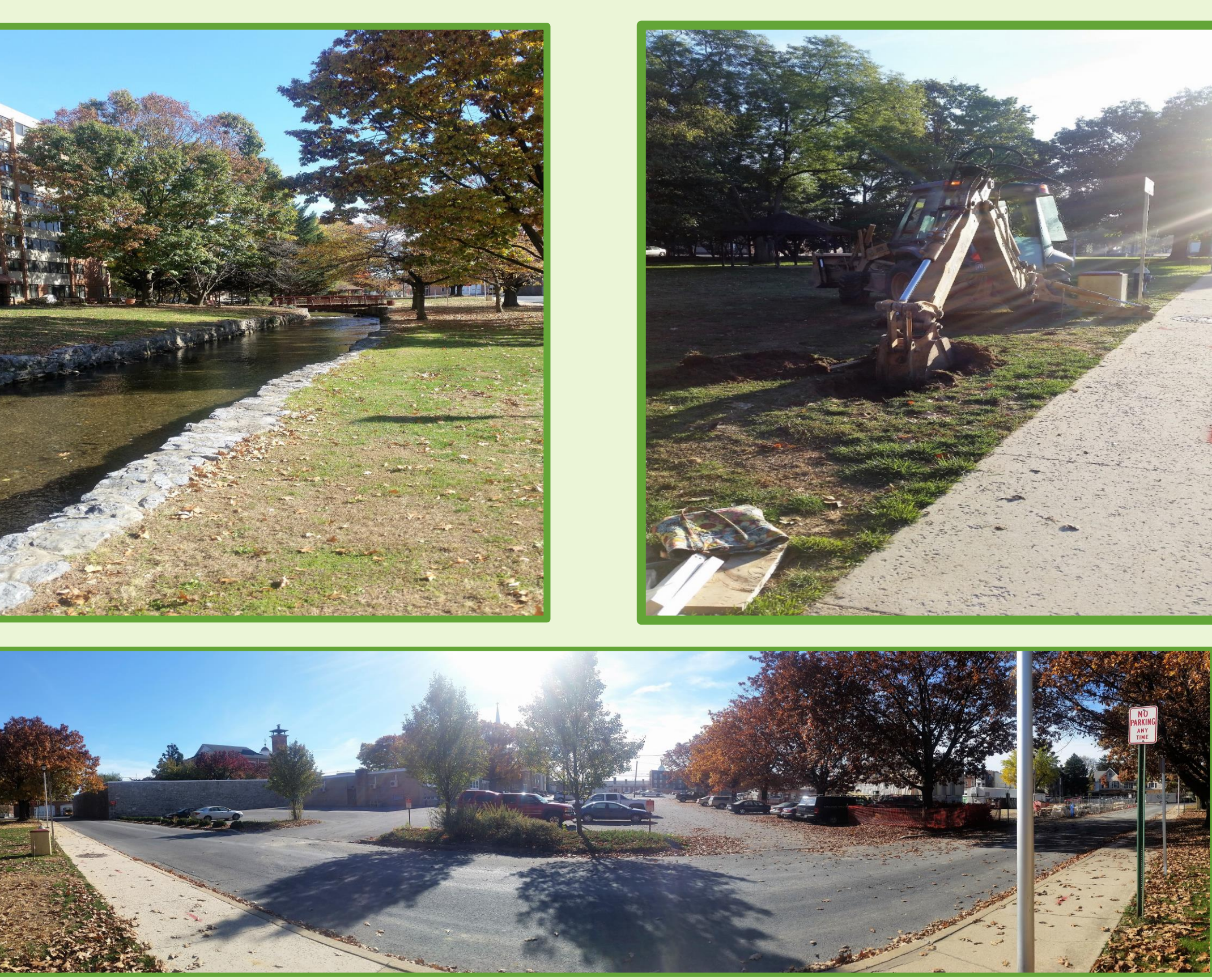
Rhodes Drive Bioretention Site
